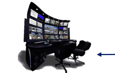
COMMAND & CONTROL CENTER MONITORING THE TOTAL NETWORK
